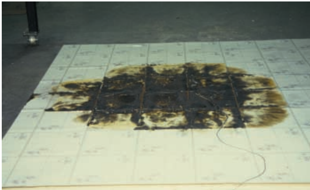
Figure 10. 1,000 mL gasoline spill fire pattern on vinyl tile floor
